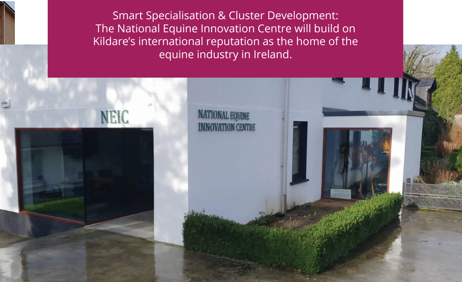
National Equine Innovation Centre @ The Irish National Stud
